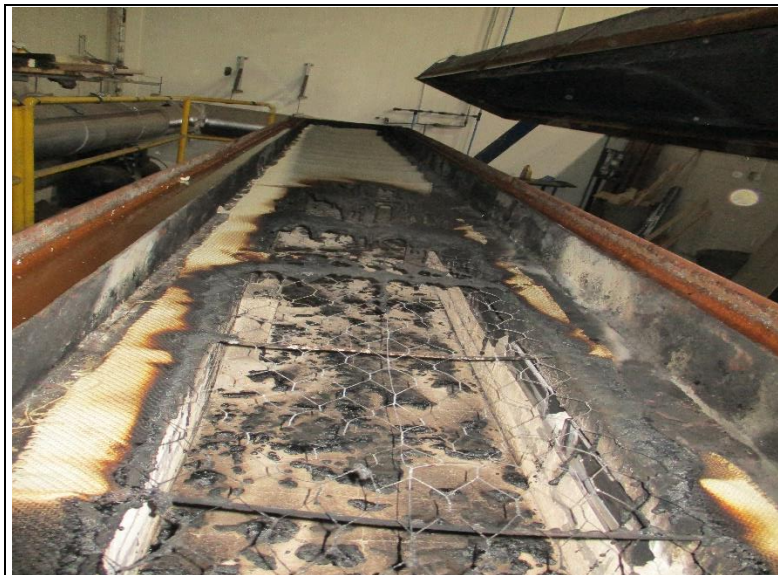
Photo No. 2 Post Test
